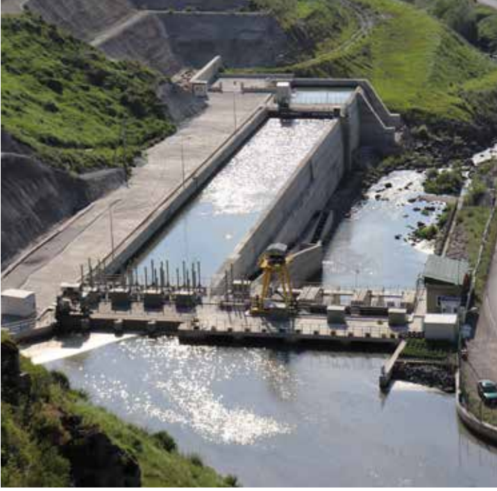
Paravani Hydroelectric Power Plant, Georgia
