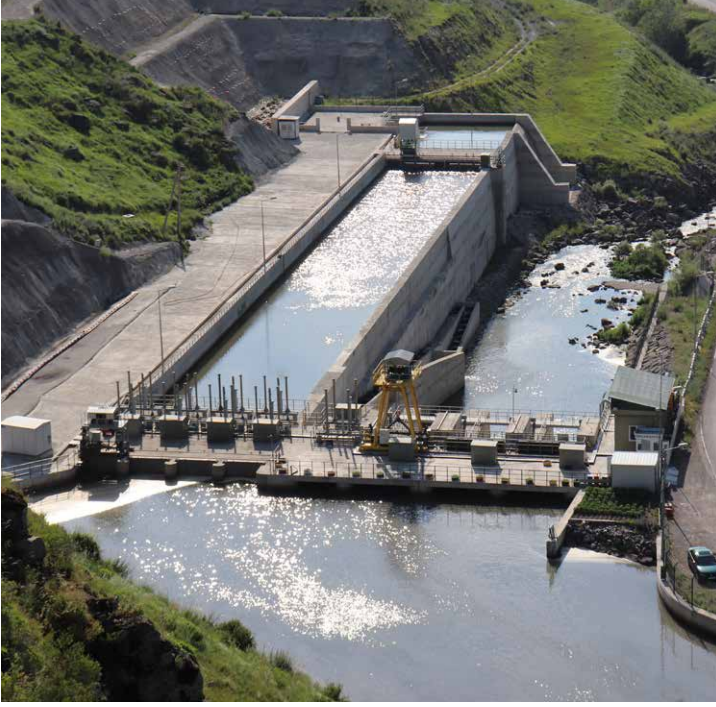
Paravani Hydroelectric Power Plant, Georgia
