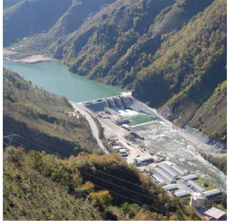
Aslancik Hydroelectric Power Plant, Giresun
