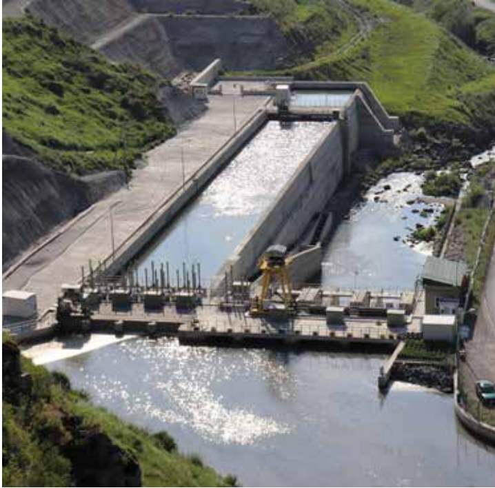
Paravani Hydroelectric Power Plant, Georgia
