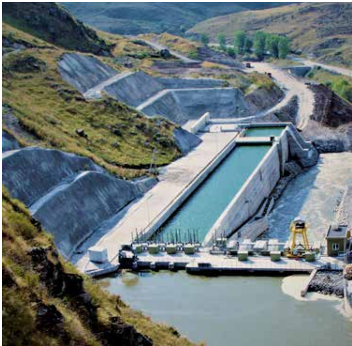
Paravani Hydroelectric Power Plant, Georgia
