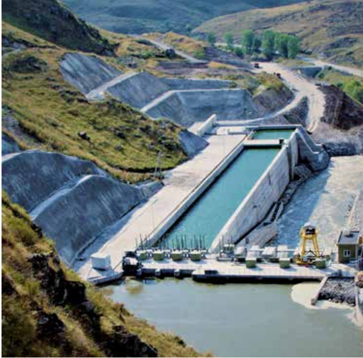
Paravani Hydroelectric Power Plant, Georgia
