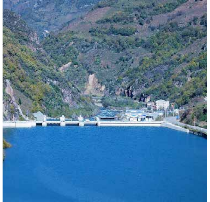
Aslancik Hydroelectric Power Plant, Giresun
