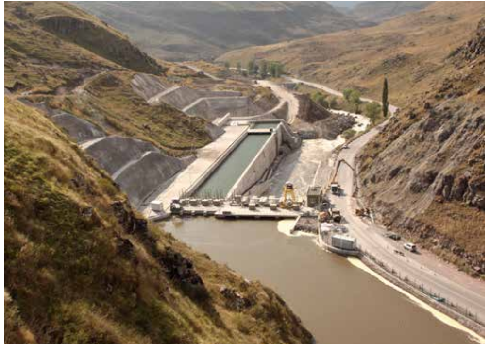
Paravani Hydroelectric Power Plant, Georgia
